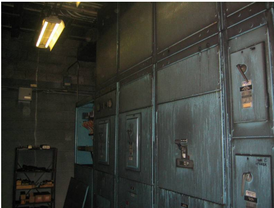
Photograph B.2 Switchgear Room, December 10, 2006
