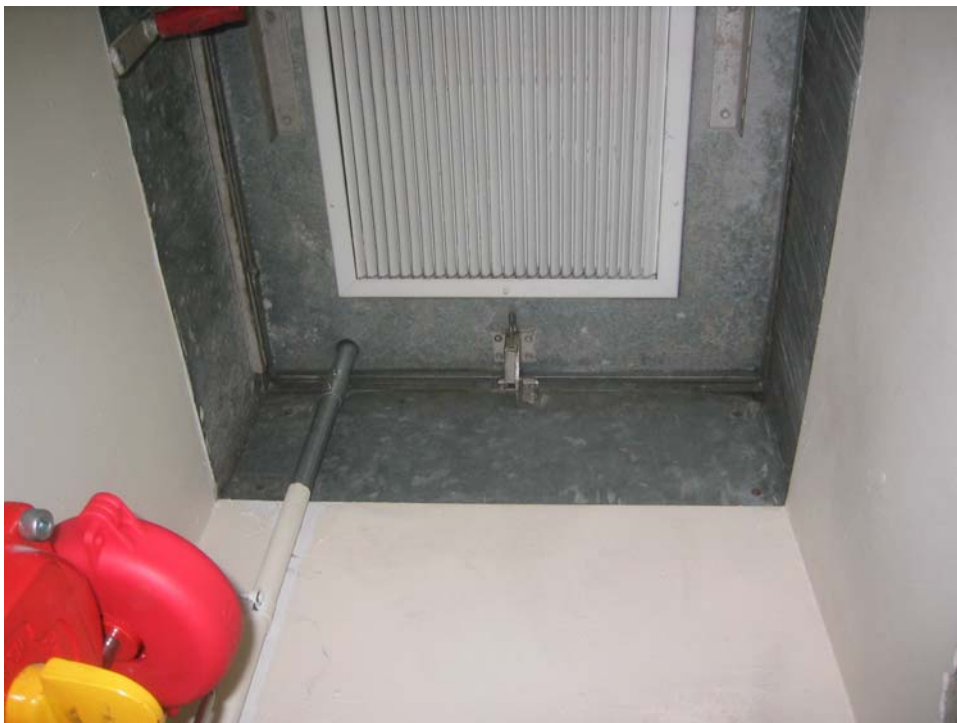
Photograph B.5 View of Stairwell Grill on Seventeenth Floor, December 10, 2006
