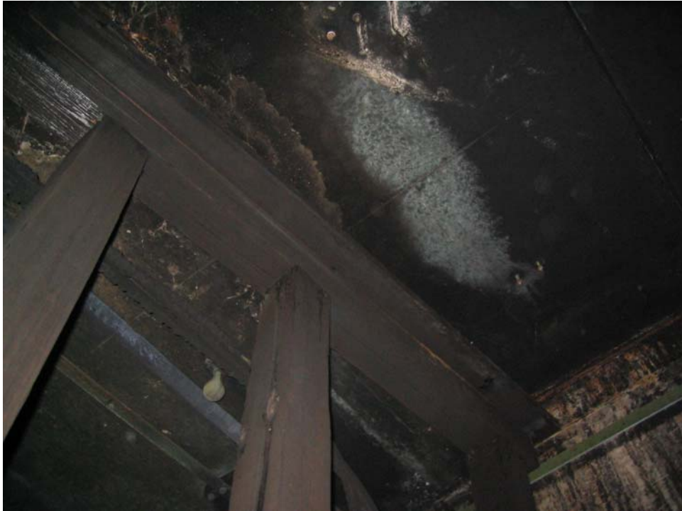
Photograph B.1 Fire-damaged Vault, December 10, 2006
